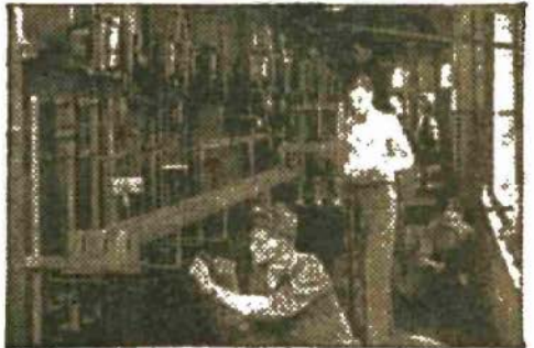
A Real Switchboard in the Coyne Shops
